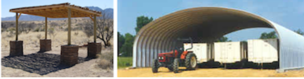
Above left: a traditional “ramada” sun-shelter in the SW United States – Right: a quonset type shelter
