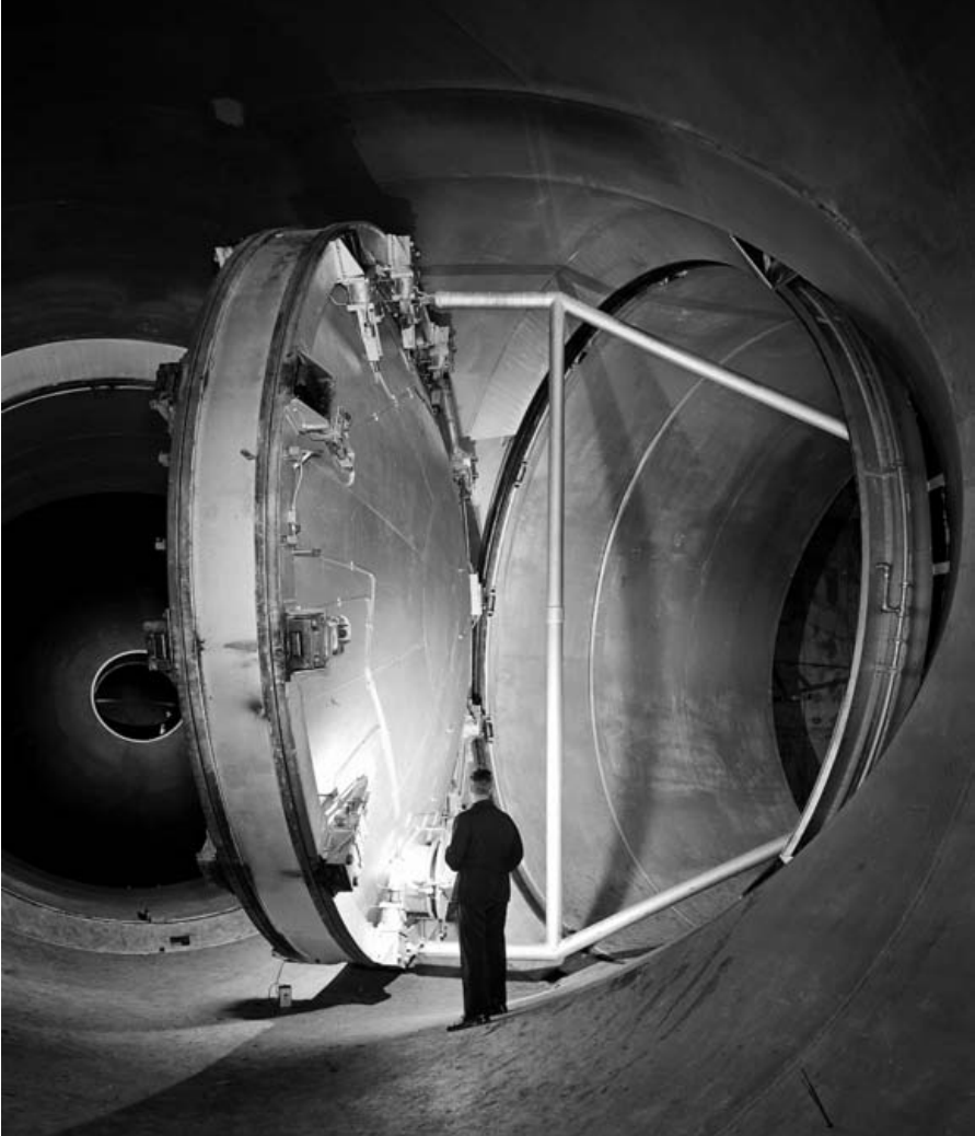
Swinging Valve for Supersonic Wind Tunnel: 1956. (NASA Lewis Research Center)
