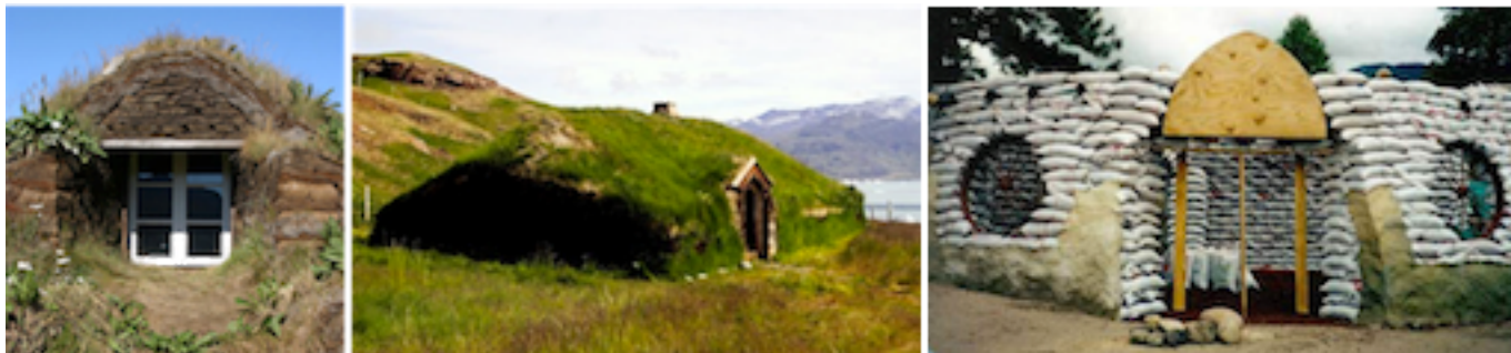
Above: Grassland Homes in tree less areas covered with insulating sod. One in Africa with sand bags
