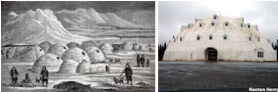
Above: Igloo Homes, and a hotel, in Arctic North America built with compressed snow blocks
