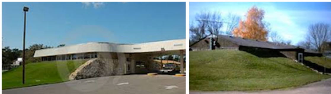
Bermed buildings: in these two, only the walls below window level are soil-insulated
